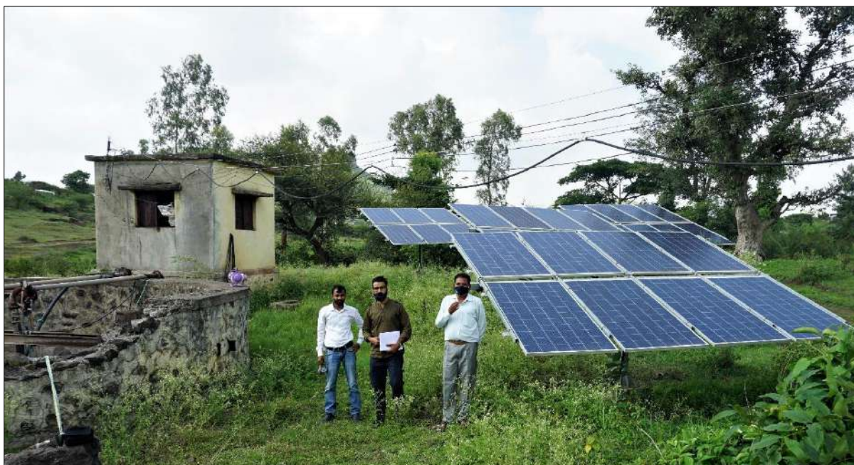
Photo 30: Solar powered unit for public drinking water well in Ashewadi
