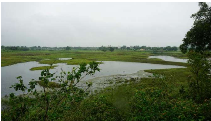
Figure 32: Heavily silted irrigation dam in Talegaon Dindori
