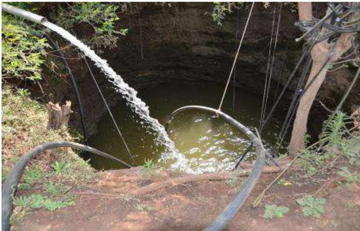
Photo 27: Water from irrigation dam being pumped in dugwell in Ashewadi village
