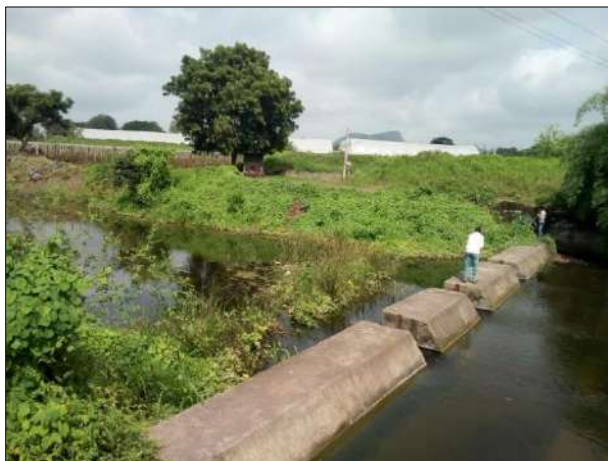
Photo 33 and 34: Team members while taking measuring the dimensions of checkdams to calculate the potential
