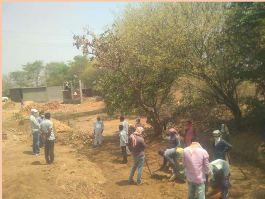
WOTR assisting in MNREGA works in Mahbubnagar district, Telangana.
